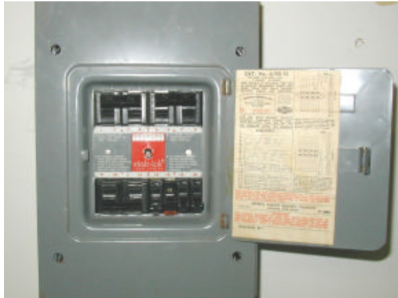
Figure 2 – Breakers that are on when down
